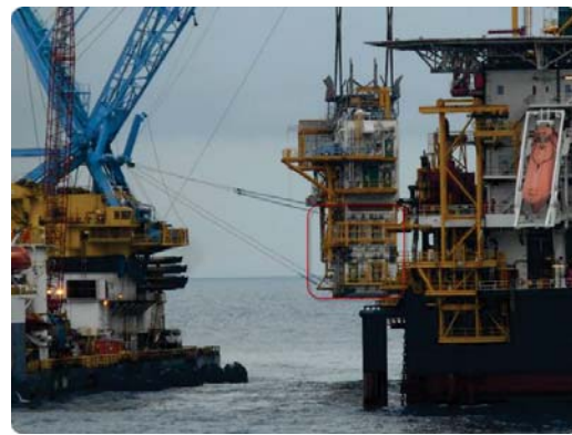
Offshore lifting to Girassol FPSO
