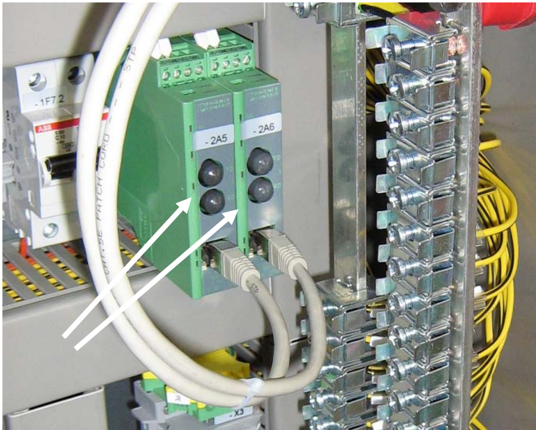
Figure 5 Fibre optic converters
