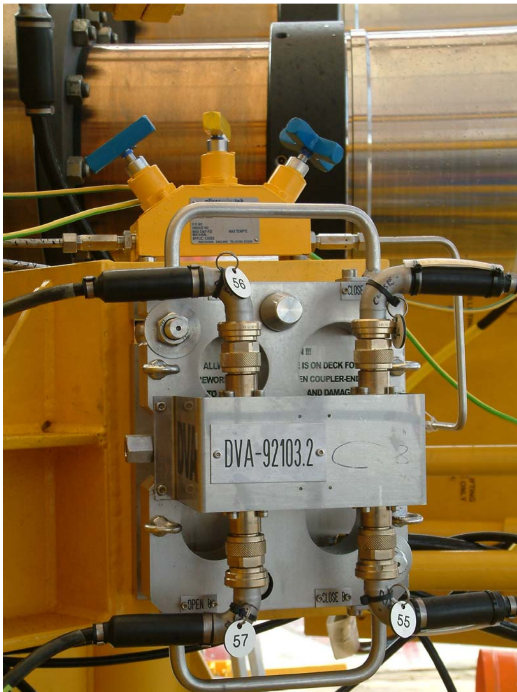
Figure: SCSSV DUMP VALVE and PROCESS / DVV / INSTRUMENT valve block
