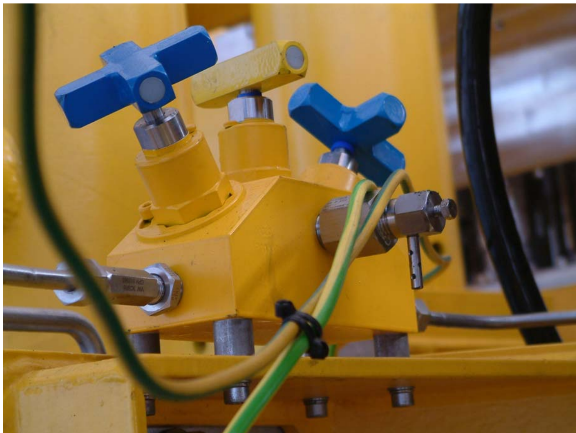
Figure: PROCESS / DVV / INSTRUMENT valve block, rear side with plug
