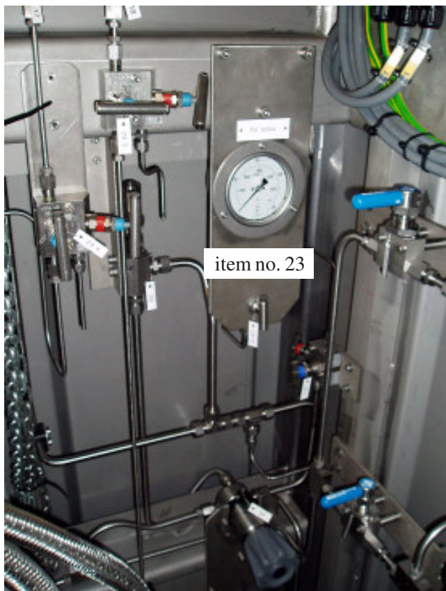
Fig. 4: ESD pilot pressure gauge, item no. 23.
