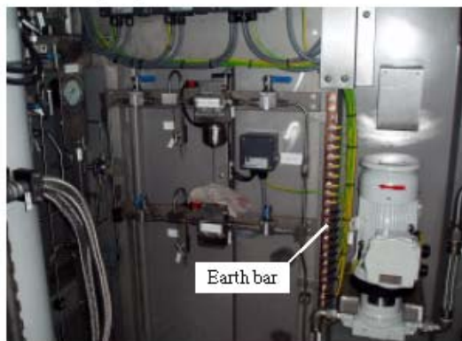
Fig. 5: Earth bar for ground connection and circulation pump.
