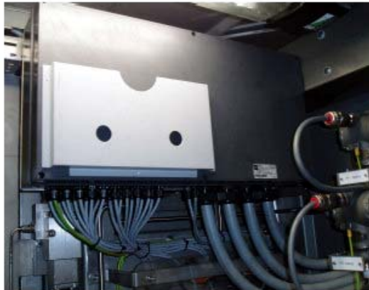
Fig. 2: Distribution box above the ESD manual valve. Junction boxes see Fig. 4.
