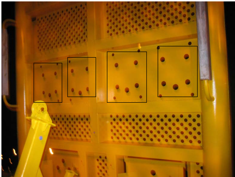
Figure: View from inside Subsea Protection Structure to 4 off SCPA mounting areas
